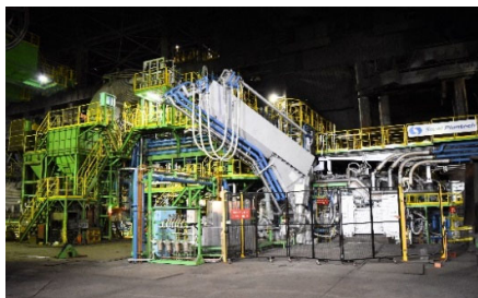
Appearance of the new electric arc furnace
